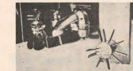
This model shows how a water wheel operates. The water hits the paddles, causing the wheel to turn.
